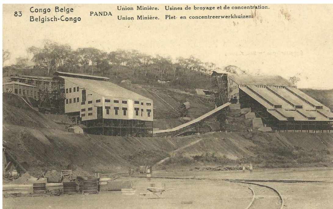
Fig. 39: Postal stationery card Stibbe type 61 of 1922, with a prepaid 15 c blue-green stamp on beige card, view 83 shows the ore mill to the left, from where a conveyor belt takes it to the concentrator on the right, which started working in late 1921. The card was written at Stanleyville on 4 October 1924 and mailed to Brussels.
