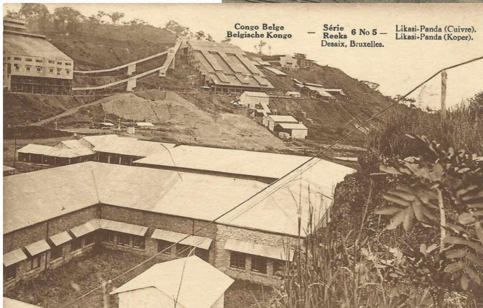
Fig. 41: This unmailed postcard no.5 in series 6 by Desaix shows the same installation from a different angle, with the experimental leaching and electrolysis plant to the right of the gravity concentrator.
