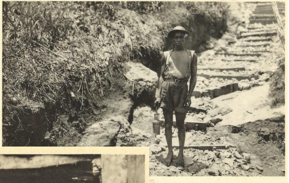
Fig. 86: The unmailed postcard above is of the Owe gold reef in the Moku area of Moto. A corridor has been driven through, with round timbers holding up beams that support the corridor roof. The clothes worn by the miner in the corridor are similar to the previous one.
