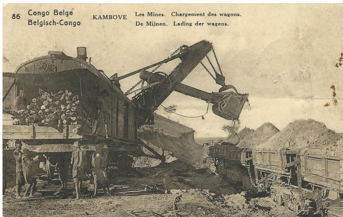
Fig. 37a: Front of postal stationery card Stibbe type 61, prepaid 15 c. blue-green on beige paper, issued in 1922. This view 86 shows a digger used to load train wagons with copper ore, to be transported to the metallurgical plant in Elisabethville. The card was written on 7 September 1928, bears additional 10, 15, 20 and 25 c definitive stamps of 1923 cancelled at Matadi on the 8th, and was mailed to the Rhineland-Palatinate.
