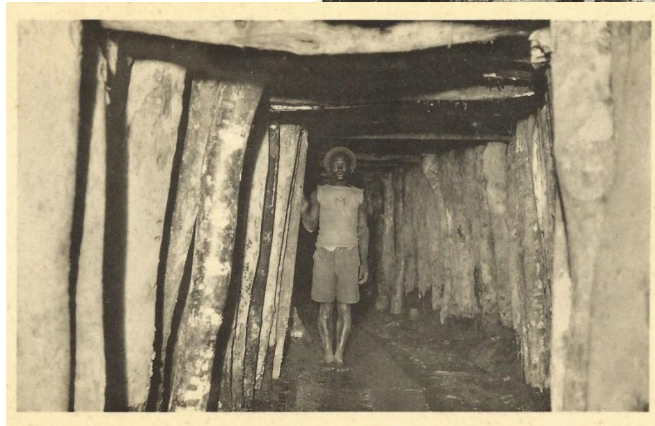
Fig. 86: The unmailed postcard above is of the Owe gold reef in the Moku area of Moto. A corridor has been driven through, with round timbers holding up beams that support the corridor roof. The clothes worn by the miner in the corridor are similar to the previous one.
